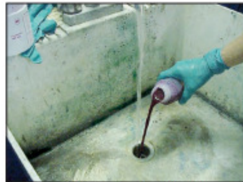
Figure 63: Dye Testing Plumbing (NEIWPCC, 2003)
